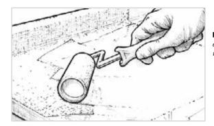
**Figure 8-22** Apply the first coat of unthickened epoxy to fill the weave of the cloth before the wet-out coat becomes completely tack free.
